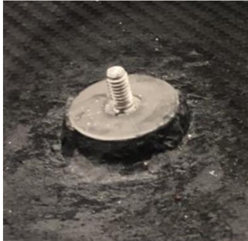
Figure 7: Previously Used Attachment Bolt
